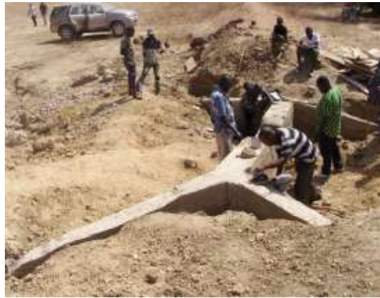
Figures 12: Spillway of a small reservoir at Apatanga in the Bongo District
