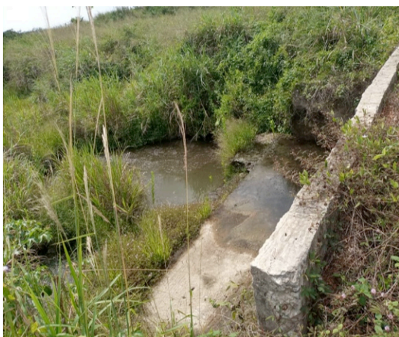
Figure 11: Weir Blocking Flow of River Asobesew by Casa de Ropa (Muni-Pomadzi Ramsar Site)
