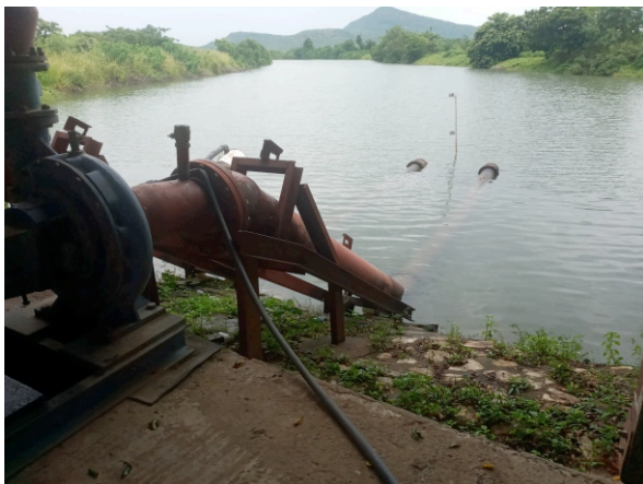
Figure 9: Site inspection of a Water Abstraction Point
