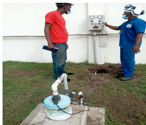
Figure 8: Inspection of GHACEM Water Facilities
