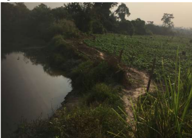
Figure 16: River bank restoration - Bia River (1)
